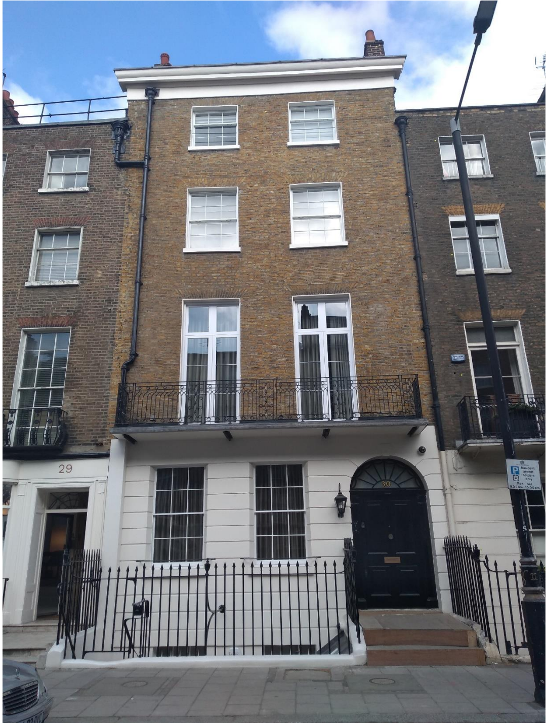
Front elevation, 30 Chapel Street SW1
